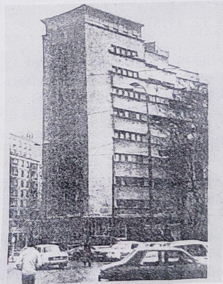
Fig.10: Apartment building with soft ground story designed and constructed prior to the 1940 Romanian earthquake.
