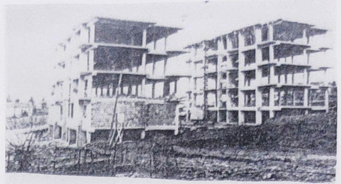
Fig. 8: Five storey eastern wing of Gemona Hospital. The second story had a discontinuity of partition walls, creating a more flexible storey
