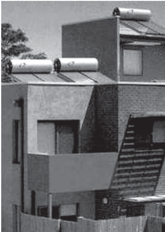
Fig. 5. Rooftop solar heater
